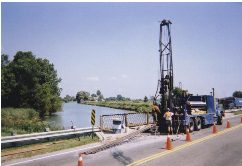
Photo 2: Drilling borehole 8 through existing bridge deck.
